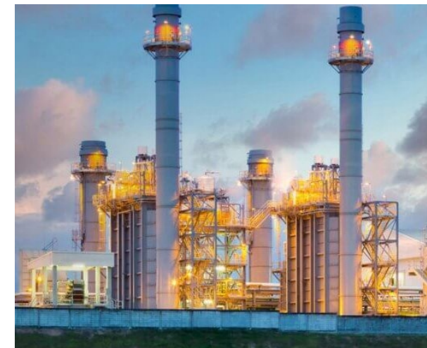
Central steam plant
